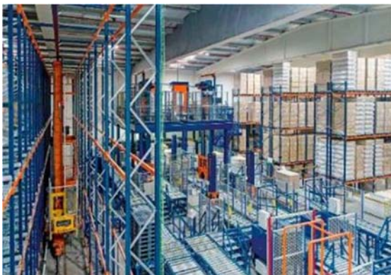
Fig. 2: Typical AS/RS warehouse conveyor and shelf system
